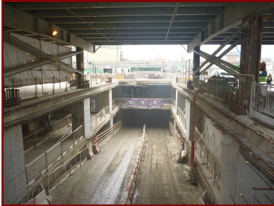
Temporary haulroad system within the construction site
