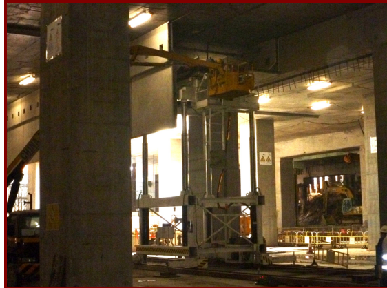
OTE installation process in place at the railway platform level
